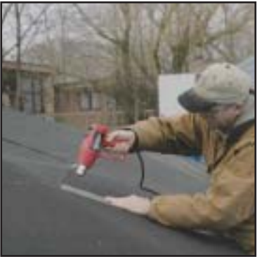
Weld Roofing Felt
